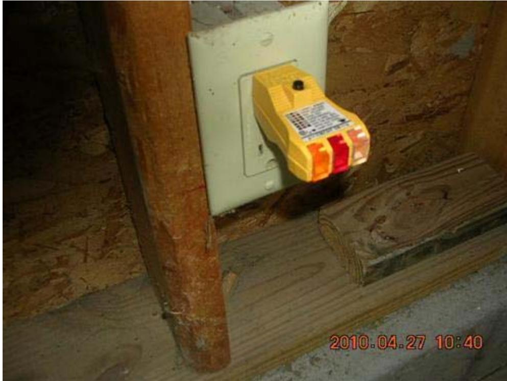
7.5 Picture 1 Incorrectly wired GFCI outlet
